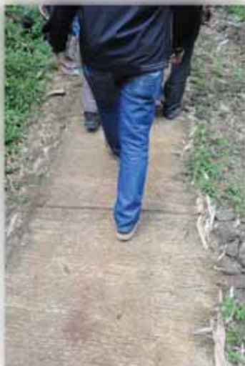
A paved path was constructed.
