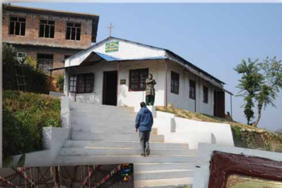
Pastor Tej ascends steps leading to the church at Dapcha. Construction was completed and the church dedicated in September 2011.
