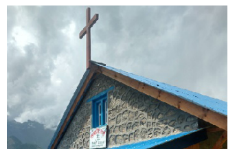
The church in Simkot, 2017
